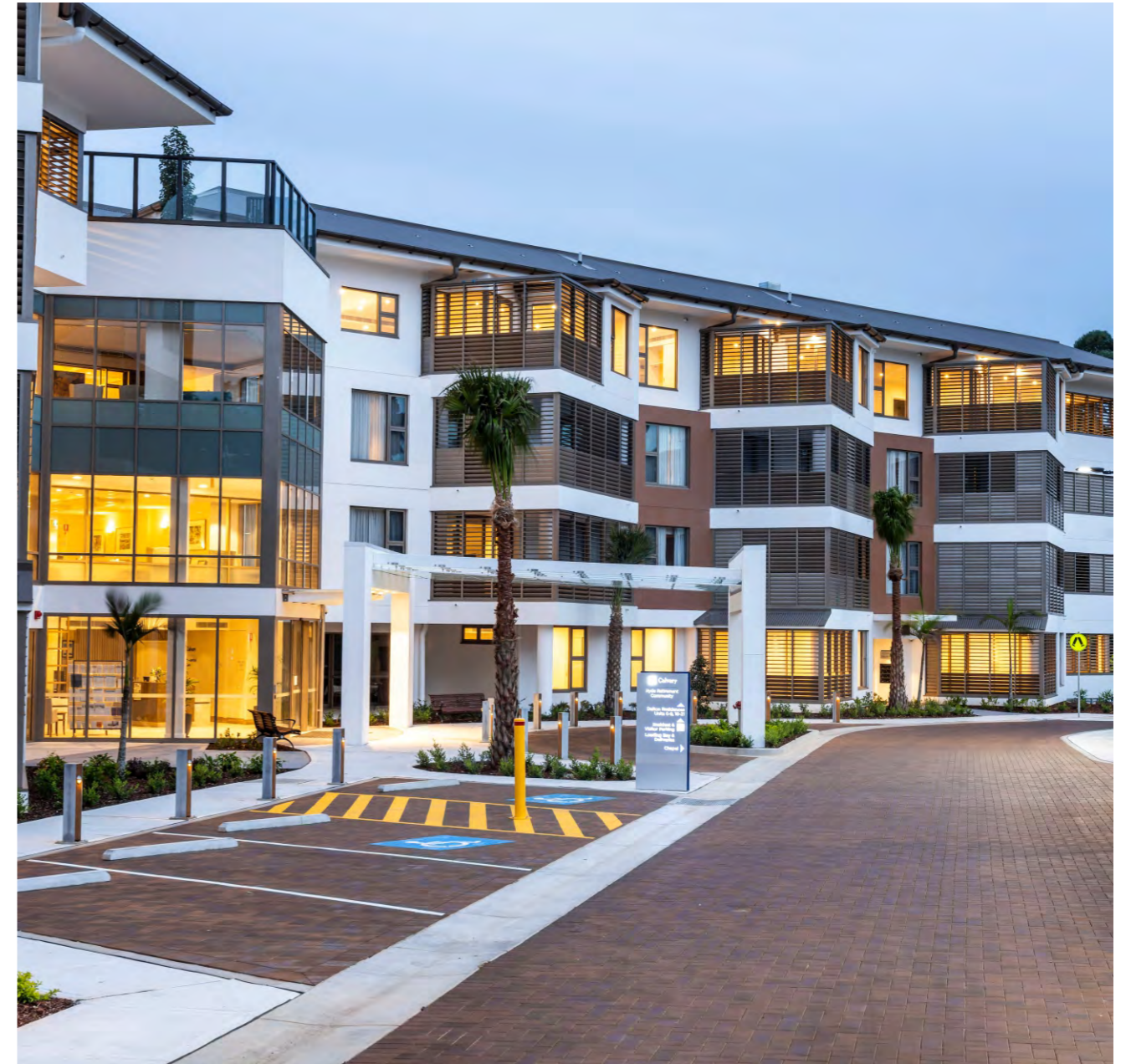
Australia Commercial Condo Project
