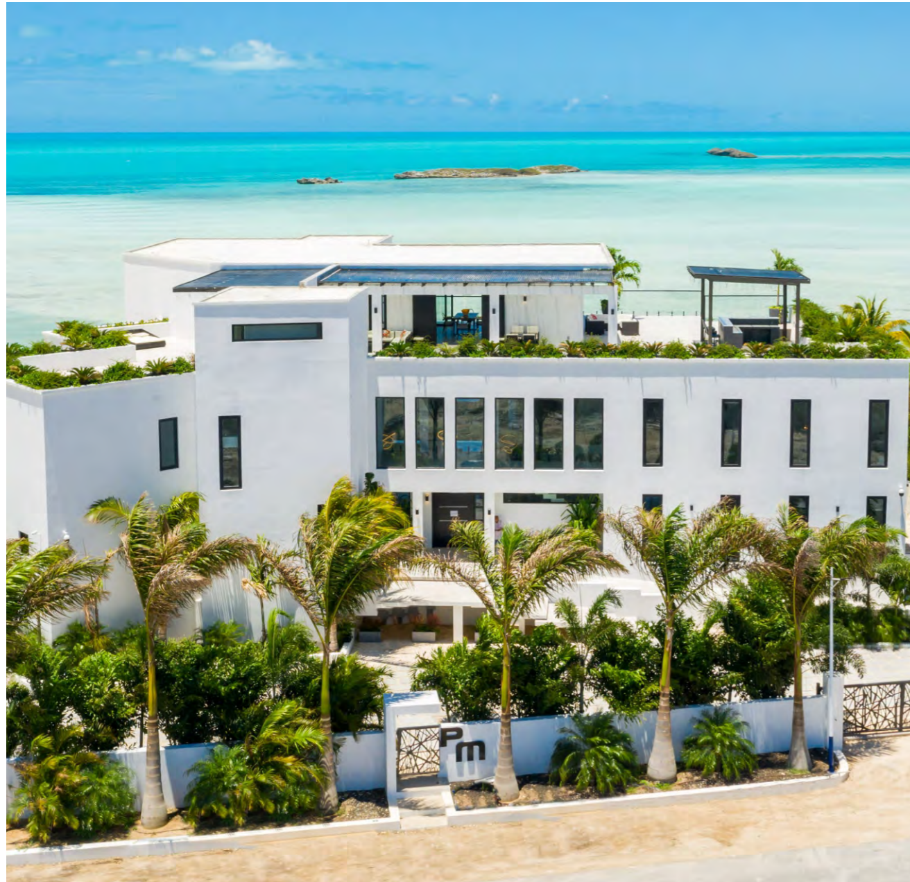
Turks Caicos Islands Residentail House Project
